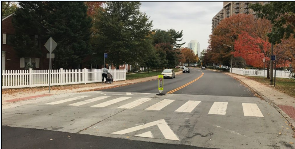
Figure 69. Photo. Illustration of a raised crosswalk.
