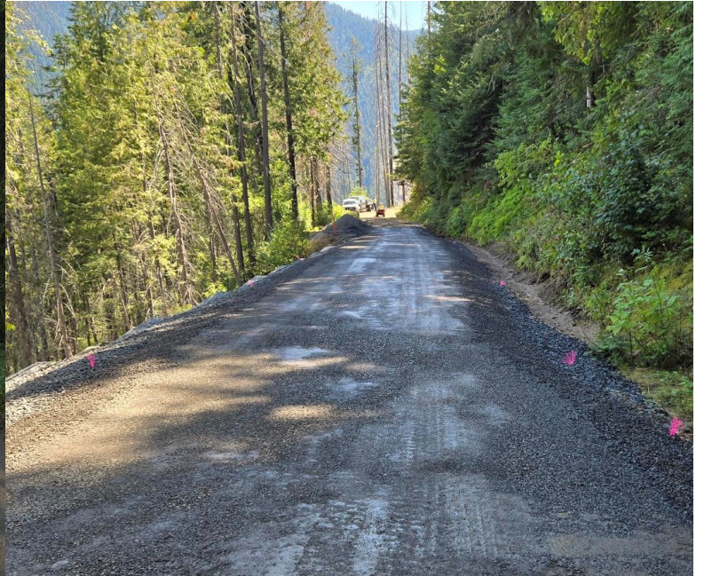
Completed roadway surface, M.P. 2.36 FSR 470
