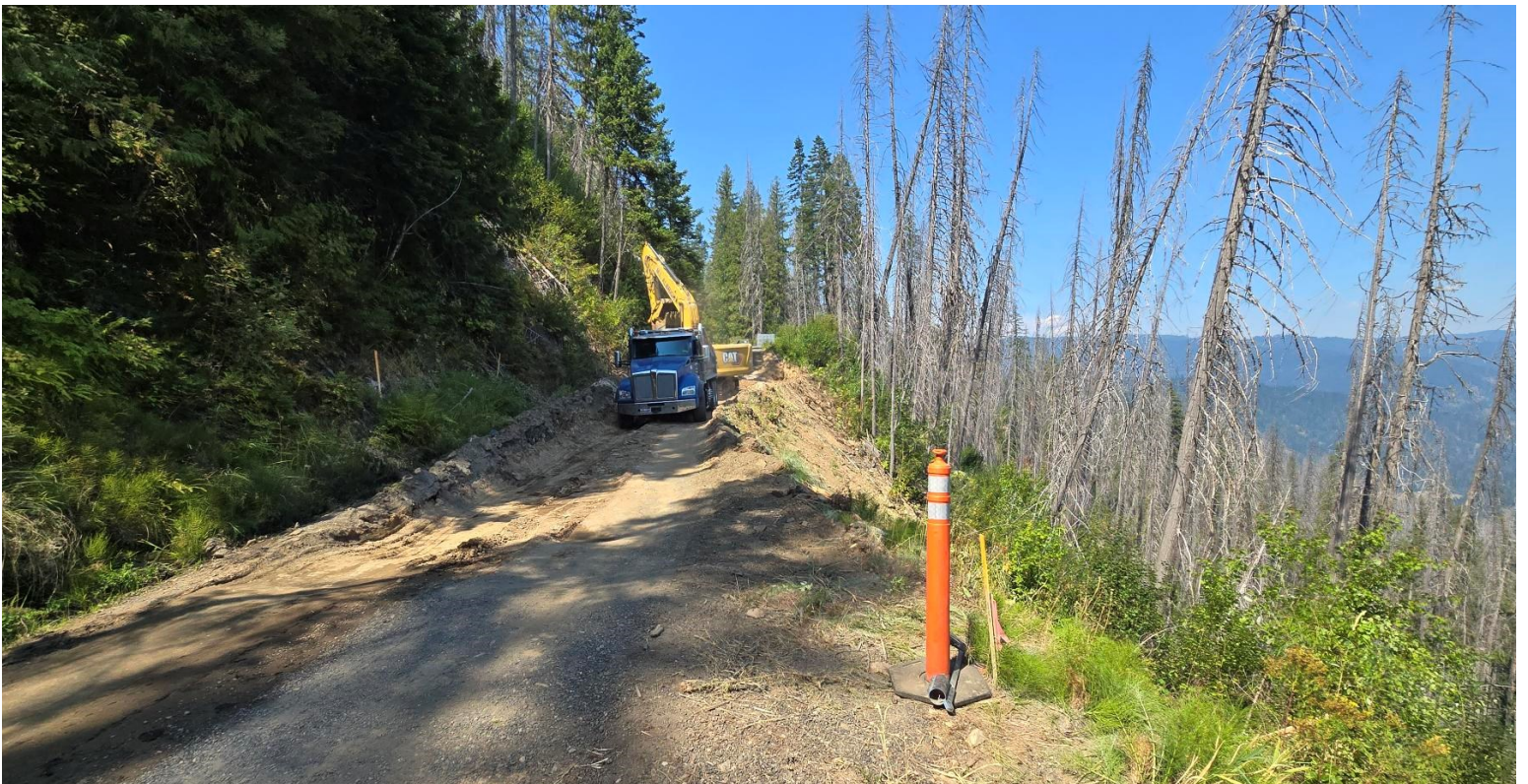
RSS Structural Excavation, M.P. 2.52 FSR 470
