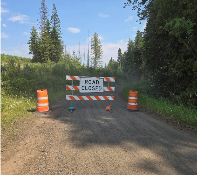
Road Closed sign, Junction FSR470 and FSR653
