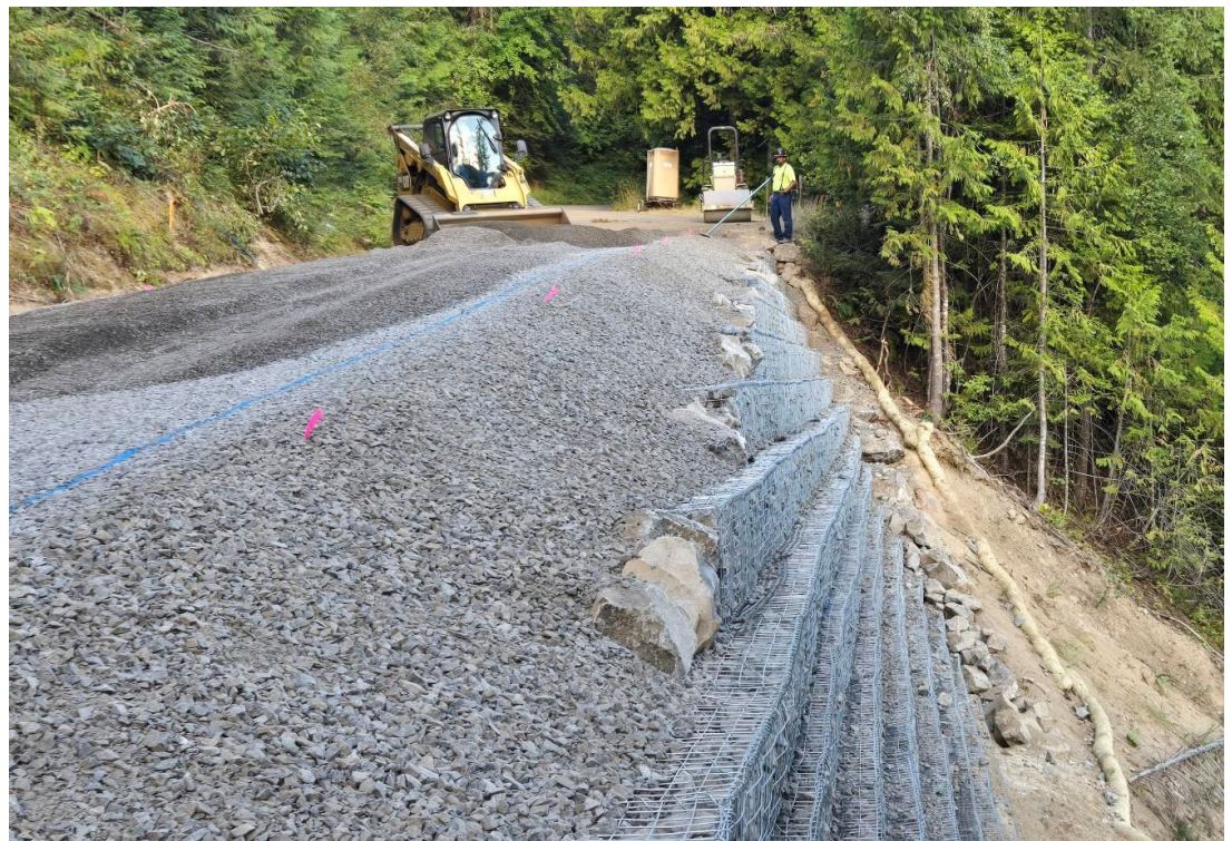
Roadway Aggregate placement M.P. 2.36 FSR 470
