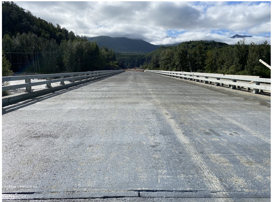
Above: Waterproof membrane applied to the new bridge.
