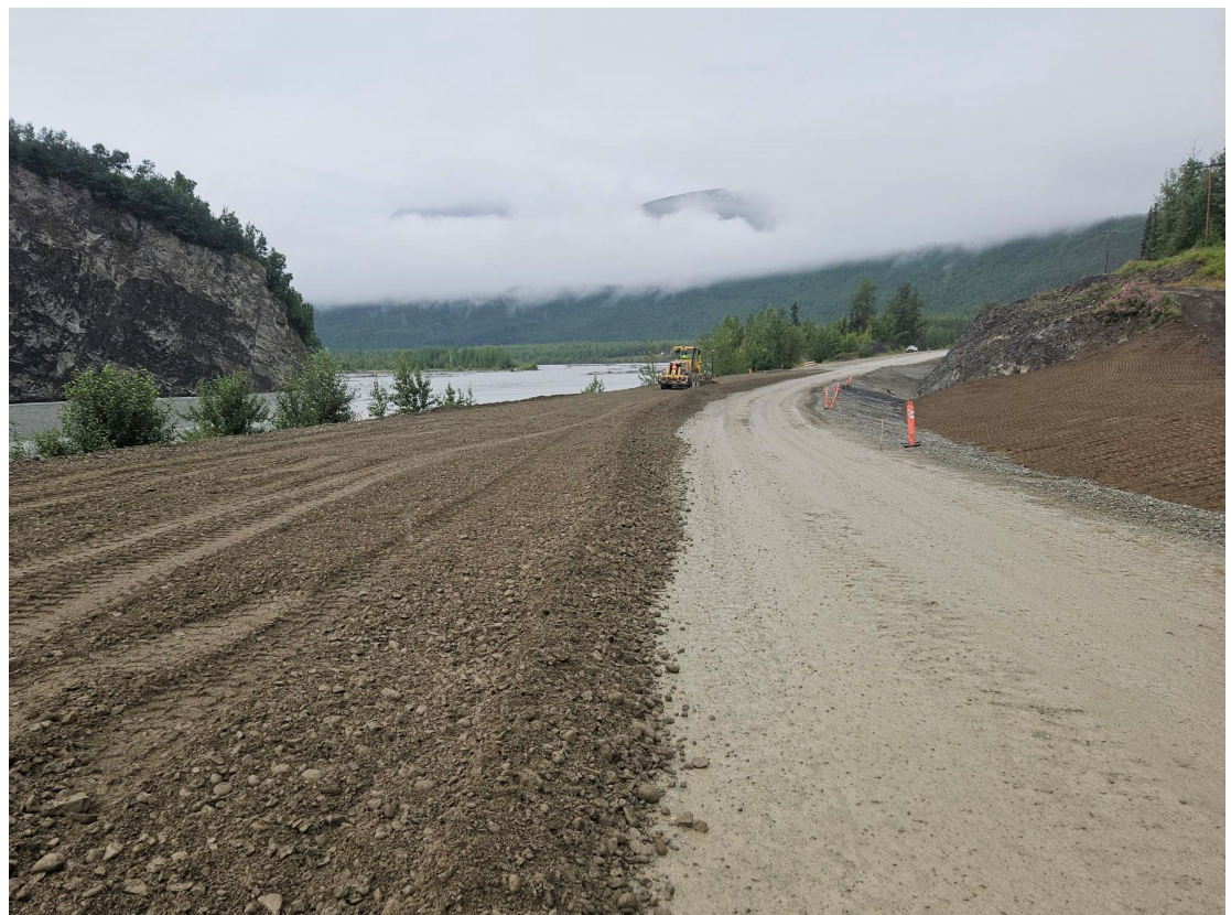
Above: Grading Select Borrow.
