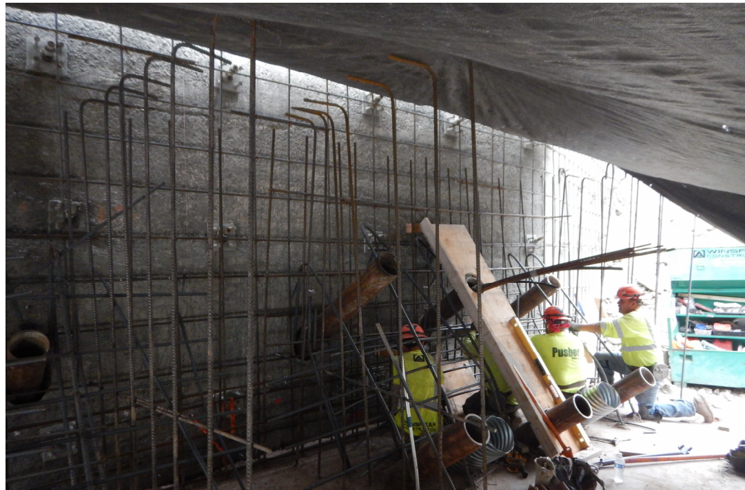
Tying reinforcing steel at Abutment 1 anchor blocks.
