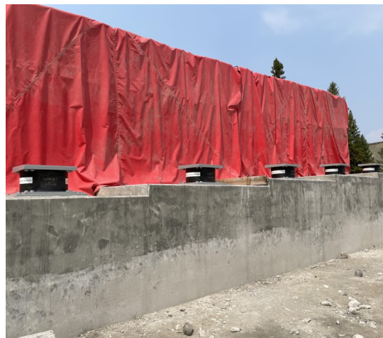
Pier 2 Cap Form Preparation
