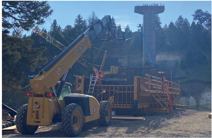
Pier 2 Cap Form Preparation
