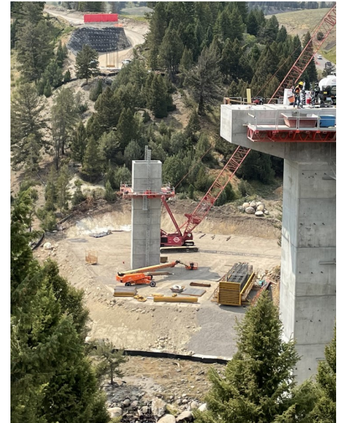
Overview of Project Site
