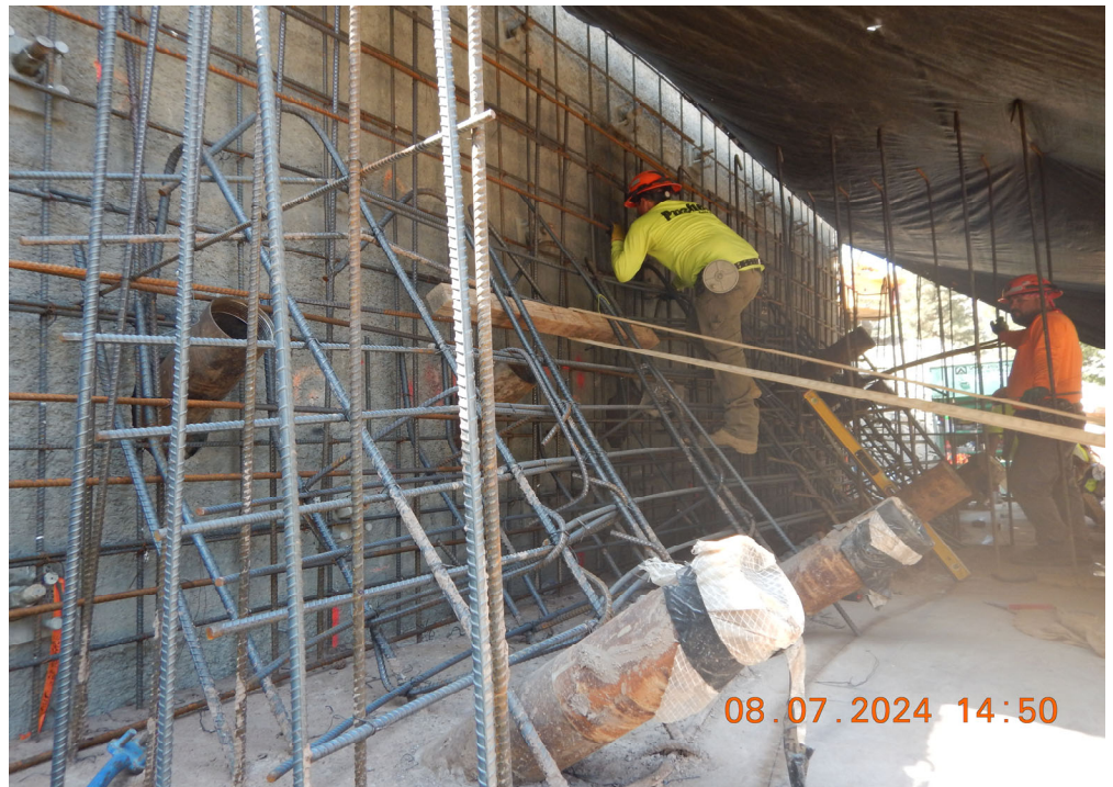
Installing and Tying Reinforcing Steel at Abutment 1 Anchor blocks.
