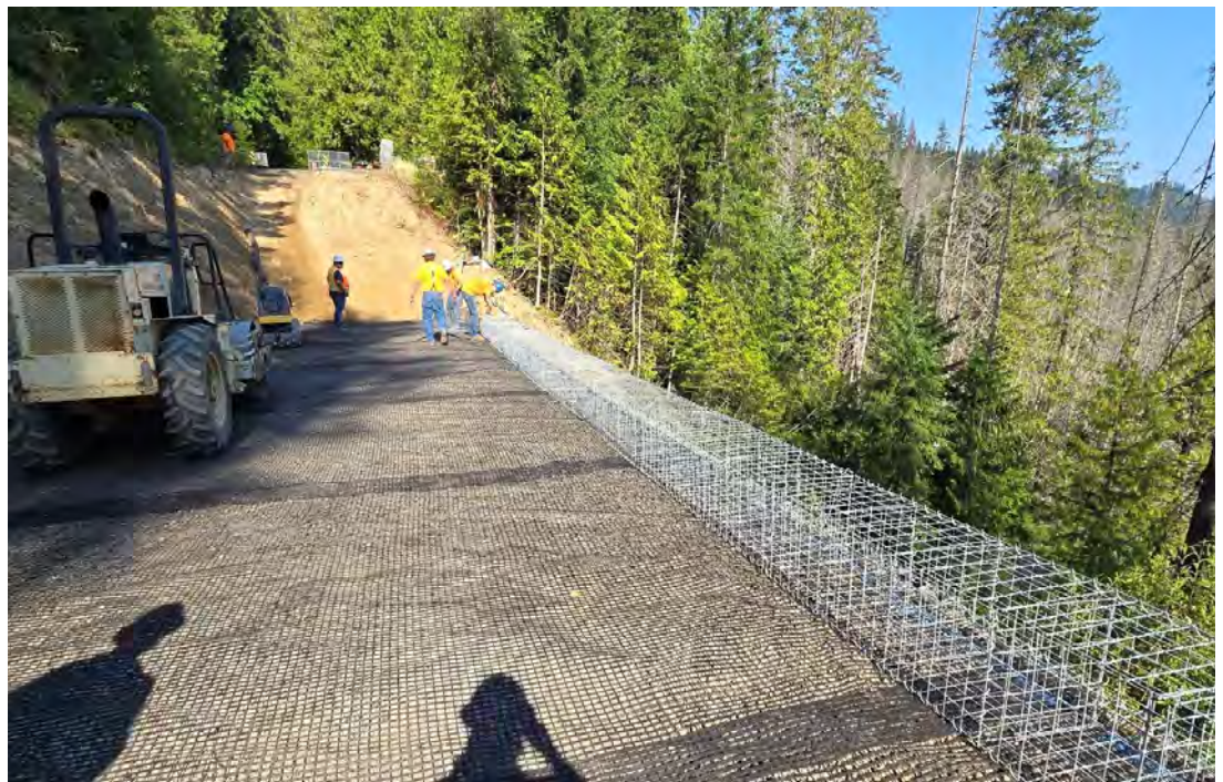
Gabion wall construction M.P. 2.36 FSR 470
