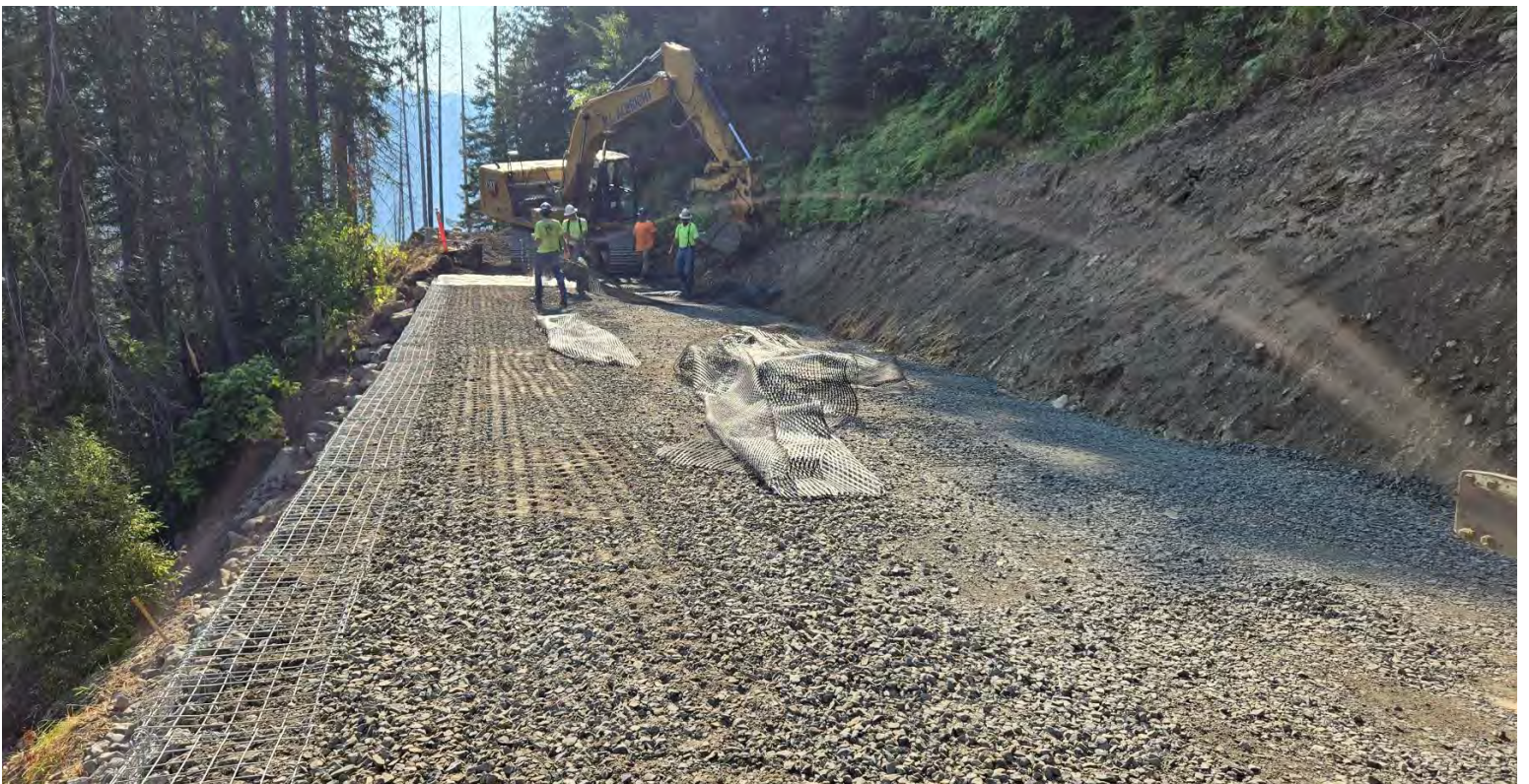
Gabion faced wall construction, M.P. 2.36 FSR 470
