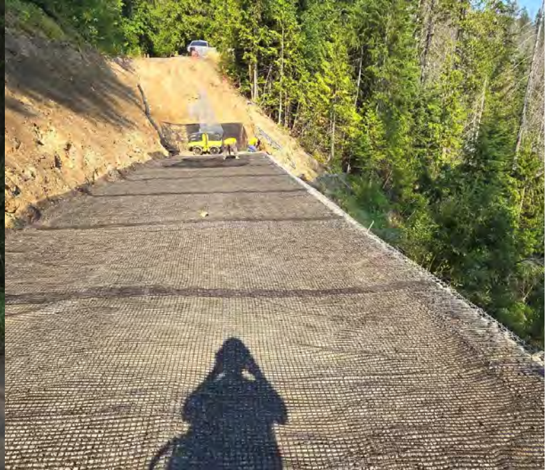
Gabion faced wall construction, M.P. 2.36 FSR 470
