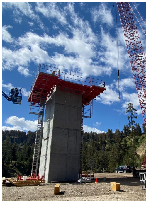
Stacking Segments at Pier 2
