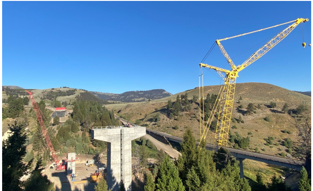
Overview of Project Site
