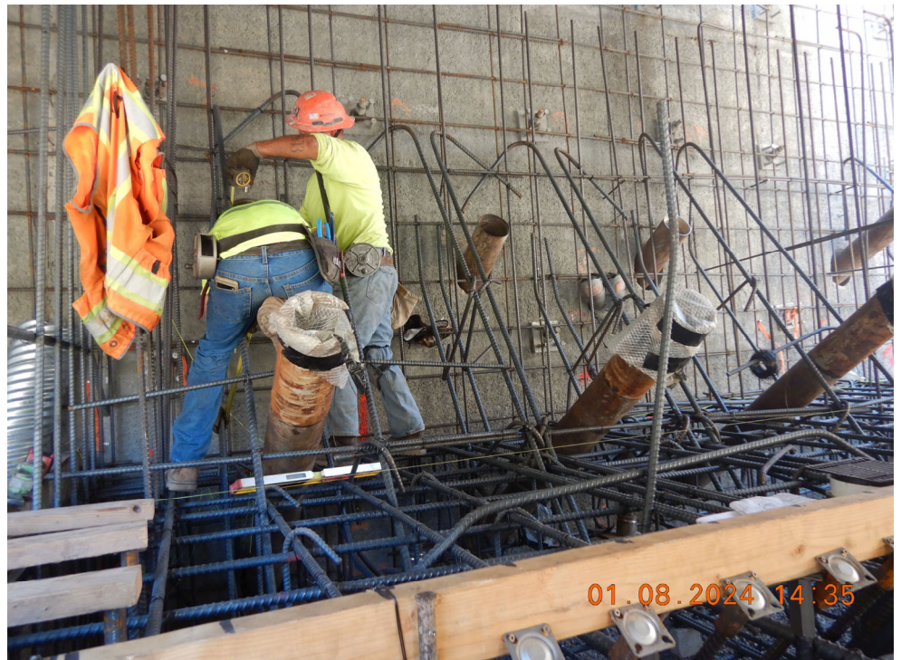
Installing and tying reinforcing bar at Abutment 1.
