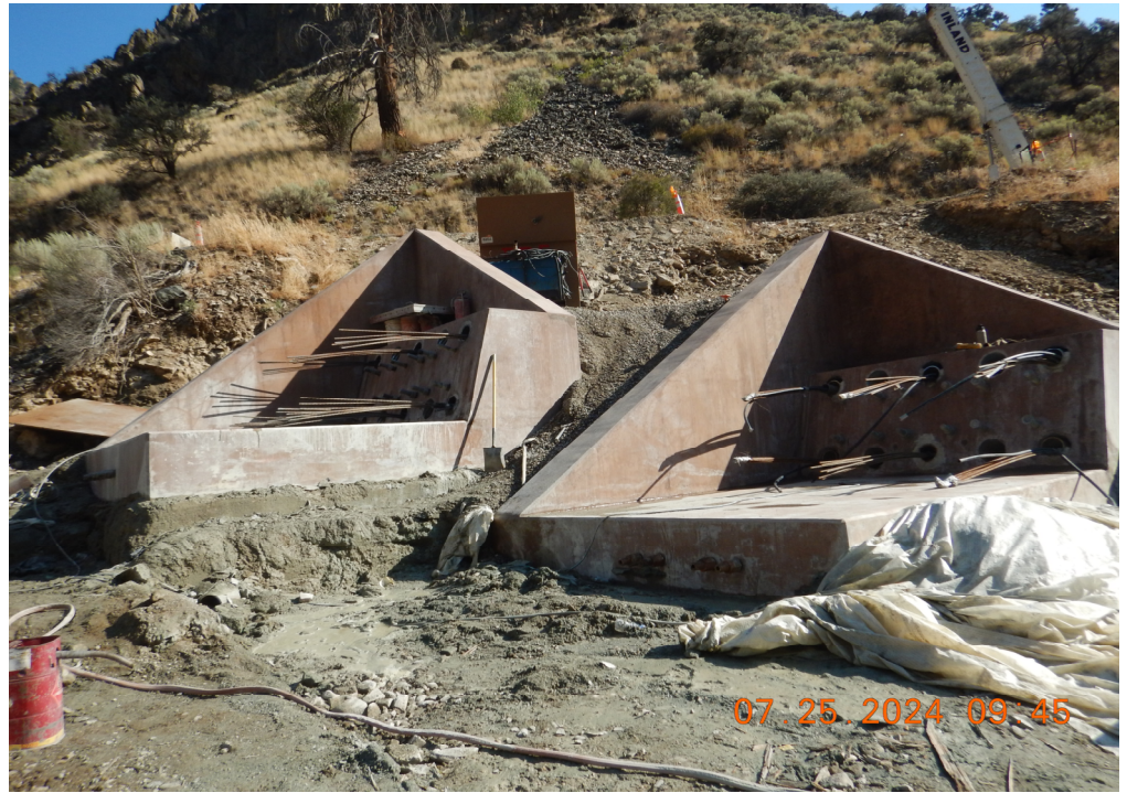
East Anchor Blocks 2A & 2B.
