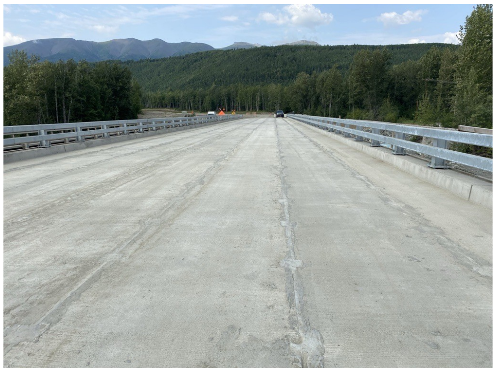
Above: New bridge deck.
