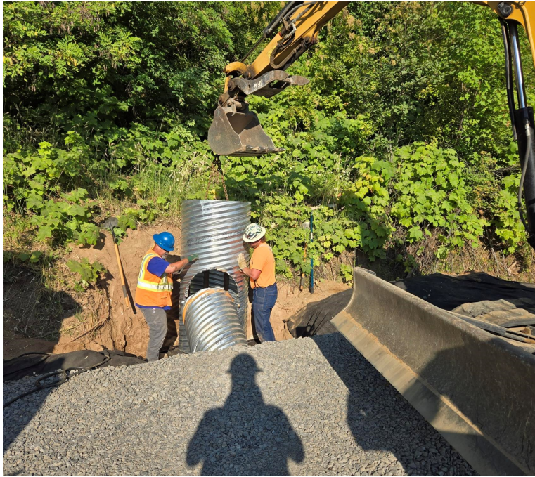
Riser Inlet installation, FSR5503
