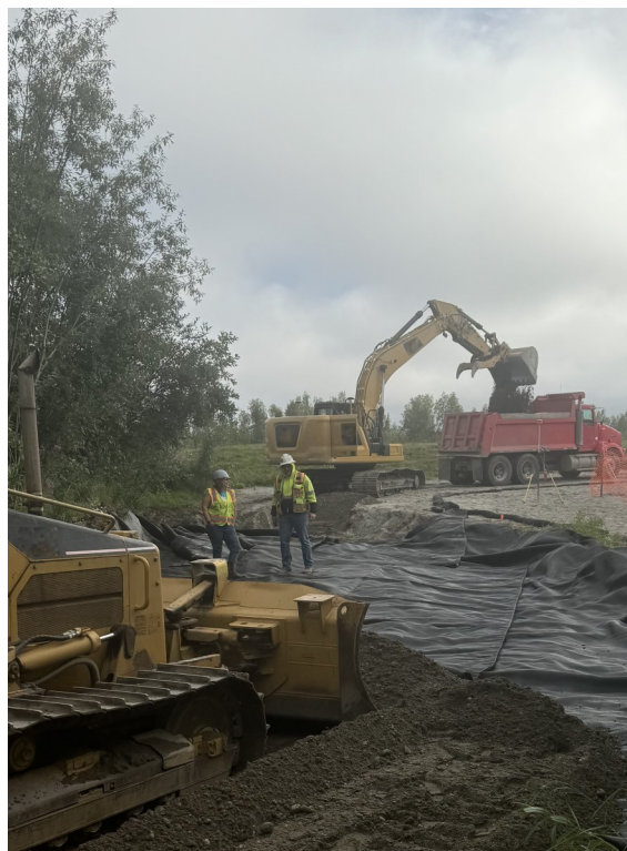
Left: Trail construction with geo fabric.
