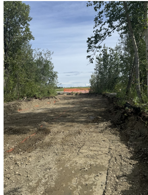
Right: Excavated trail.
