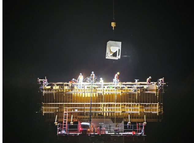
Formwork and shoring of Pier 3 End Cap
