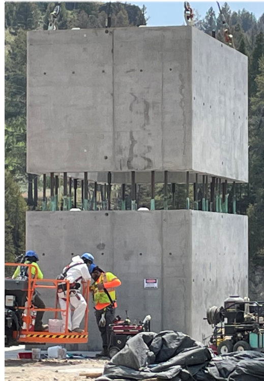
Placement of Pier 2 segment
