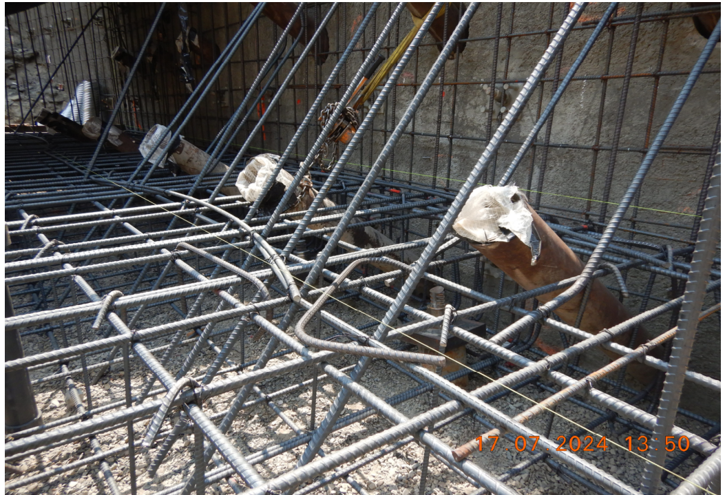
Reinforcing steel Abutment 1 and Anchor Blocks.
