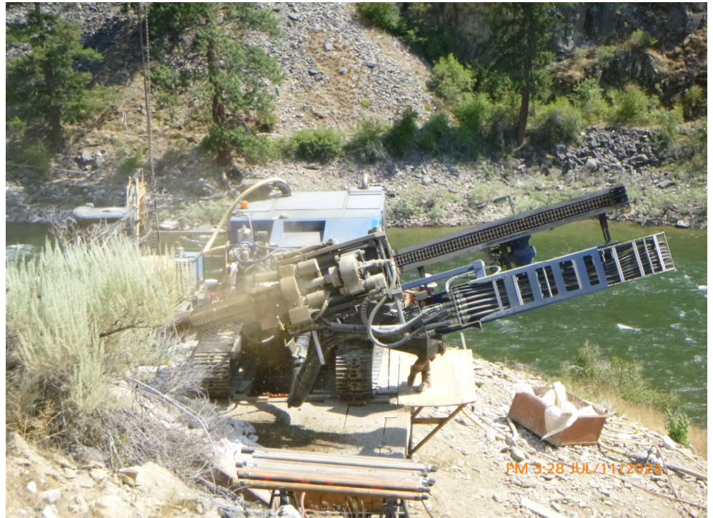
Drilling permanent ground anchors at EAB 2A
