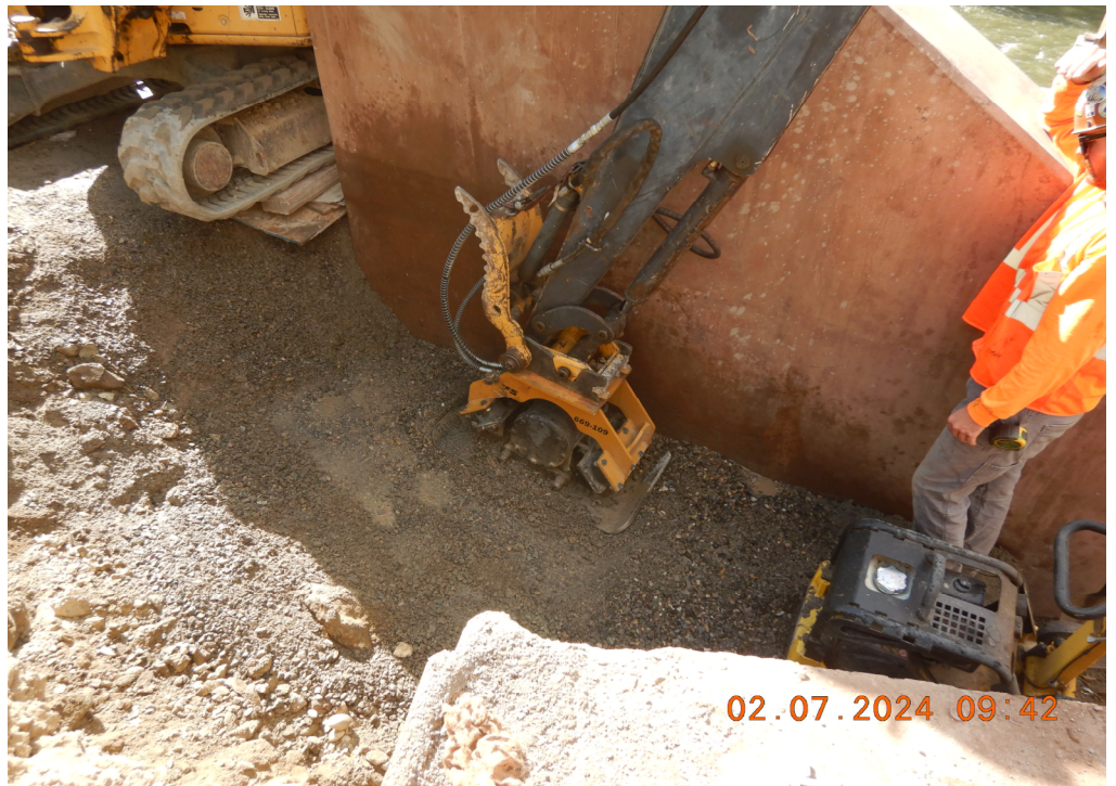
Select Backfill and compaction EAB 2B.
