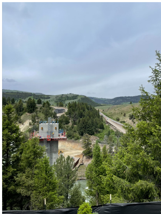
Pier 3 Pre-cast segments
