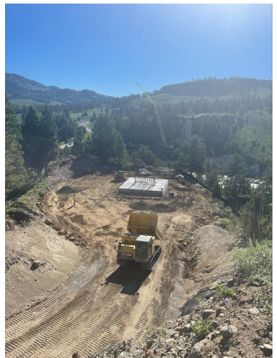
Pier 1 Backfill
