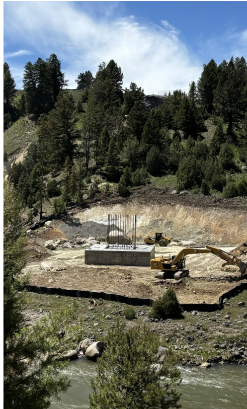
Pier Two Footing View from Pier Three
