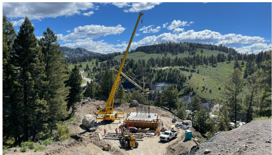
Pier One Forms Being Stripped
