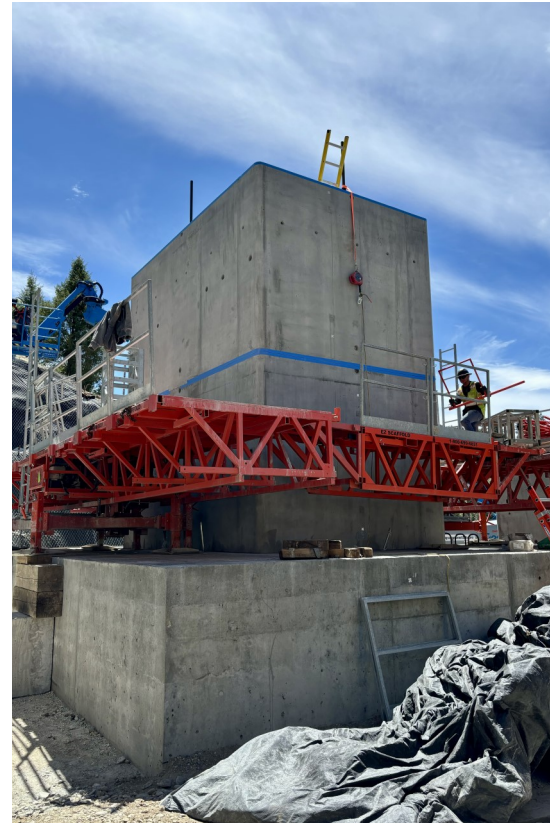
Pier Three with Two Segments Stacked
