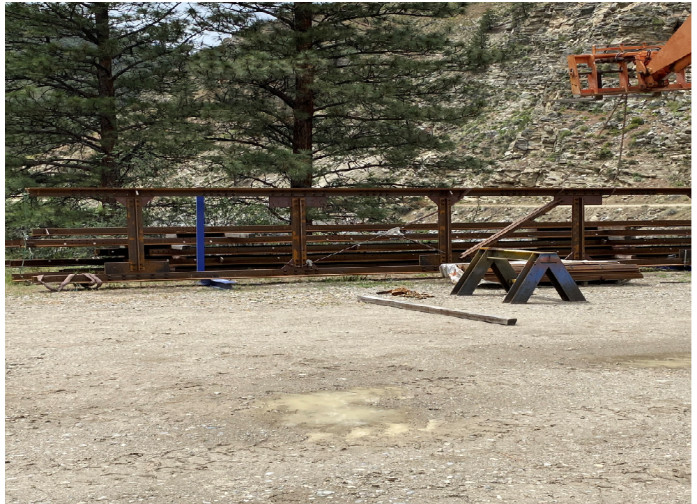
Assembly of bridge trusses
