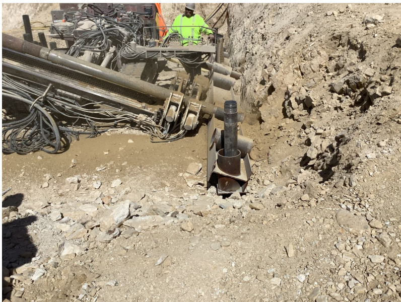
Drilling for the micropiles at the east abutment location.
