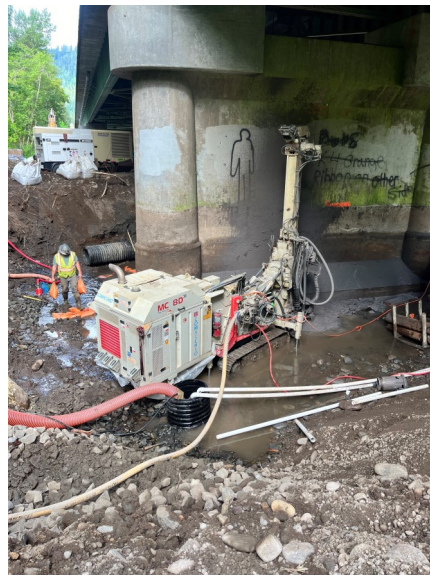
6-5-24 Barnard Pier 5 Micropiles
