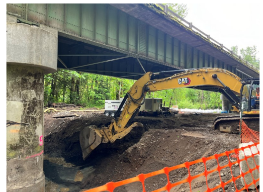
6-3-24 Barnard Pier 5 Excavation
