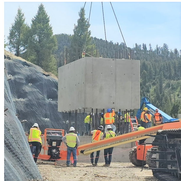
Placement of 1st pier segment, Pier 3
