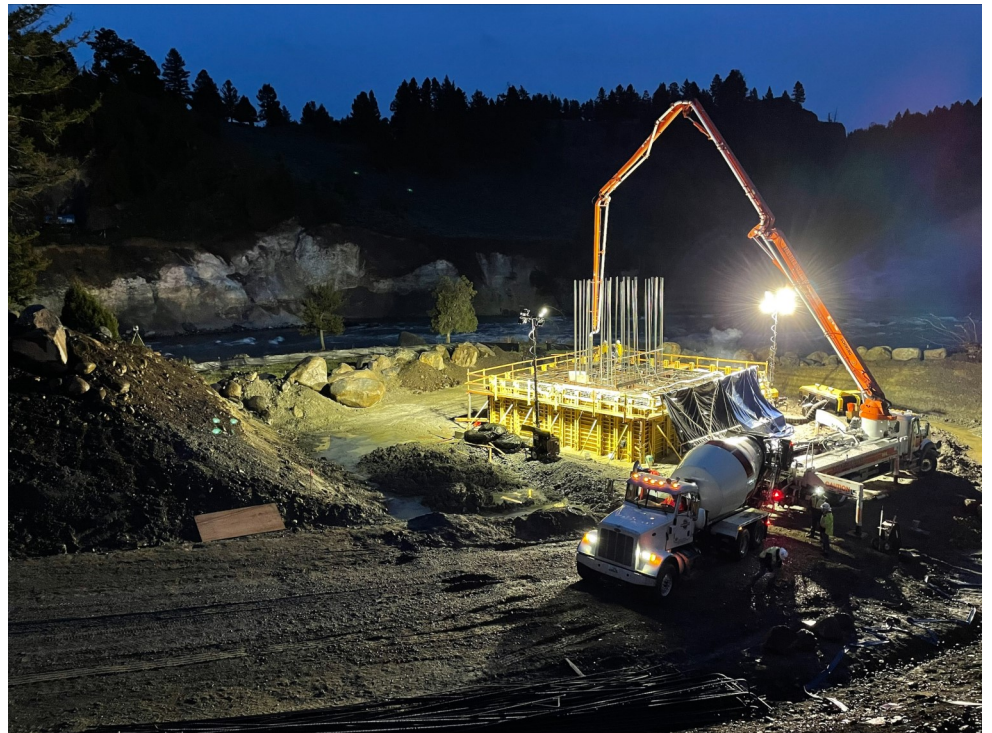
Concrete Placement at Pier 2 Footing
