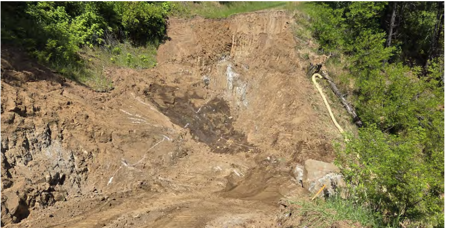
Completed Slide Excavation, FSR 5503 M.P. 1.28
