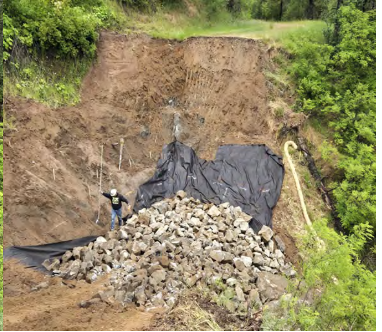
Special Rock Embankment, FSR 5503 M.P. 1.27
