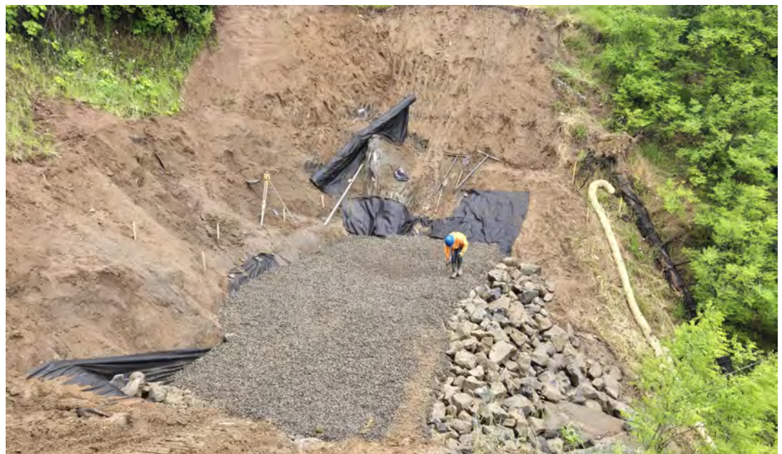
Special Rock Embankment and leveling course at FSR5503.
