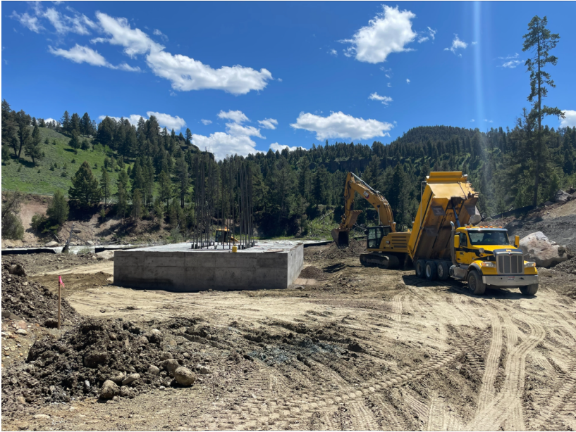
Backfill Pier 2 Footing
