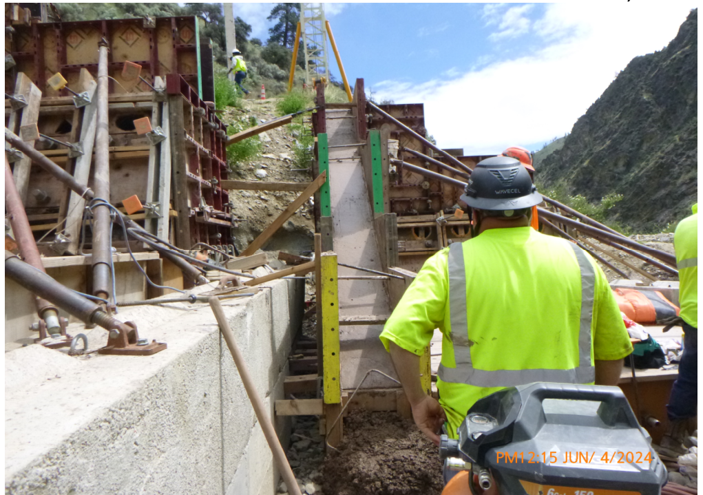
EAB 2A & 2B concrete wall placement
