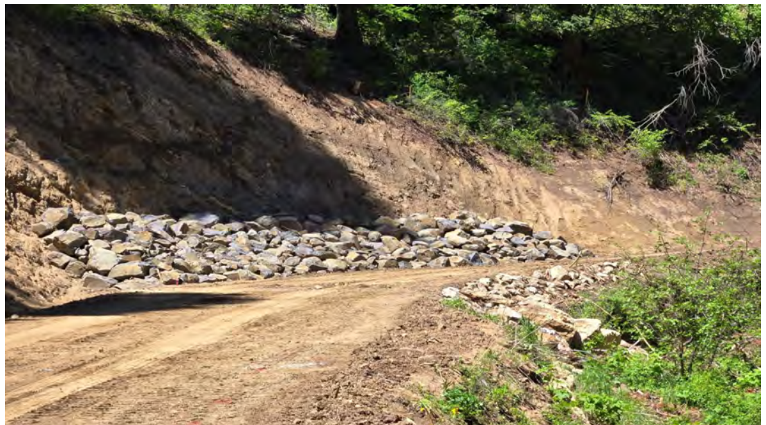
Rock buttress and shoulder stabilization FSR354 M.P. 13.6
