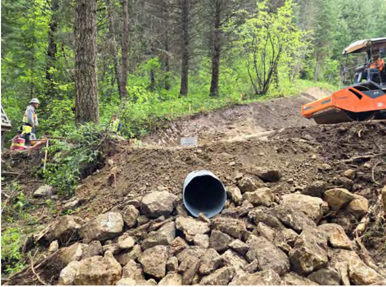
24-inch culvert install M.P. 13.6 FSR354
