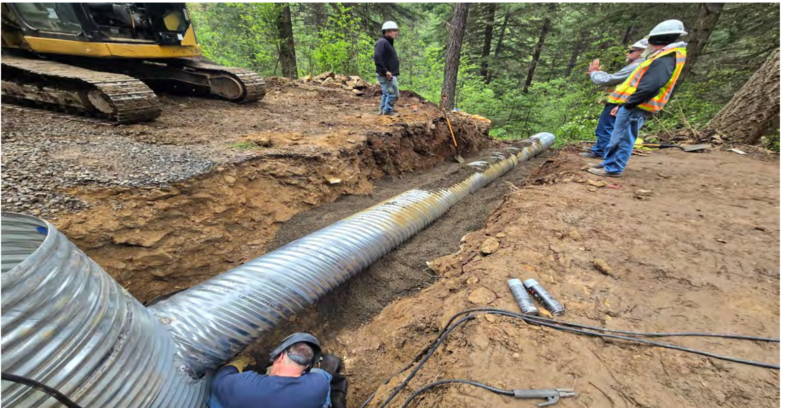
Culvert installation FSR 354 M.P. 13.6
