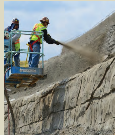
Soil nail wall example
