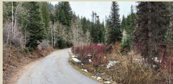
Steep slopes and creek adjacent to the road
