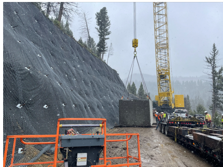
Pre-cast Segment Delivery
