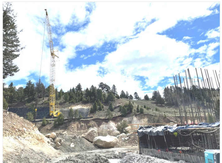
Crane Being Erected at Pier 3
