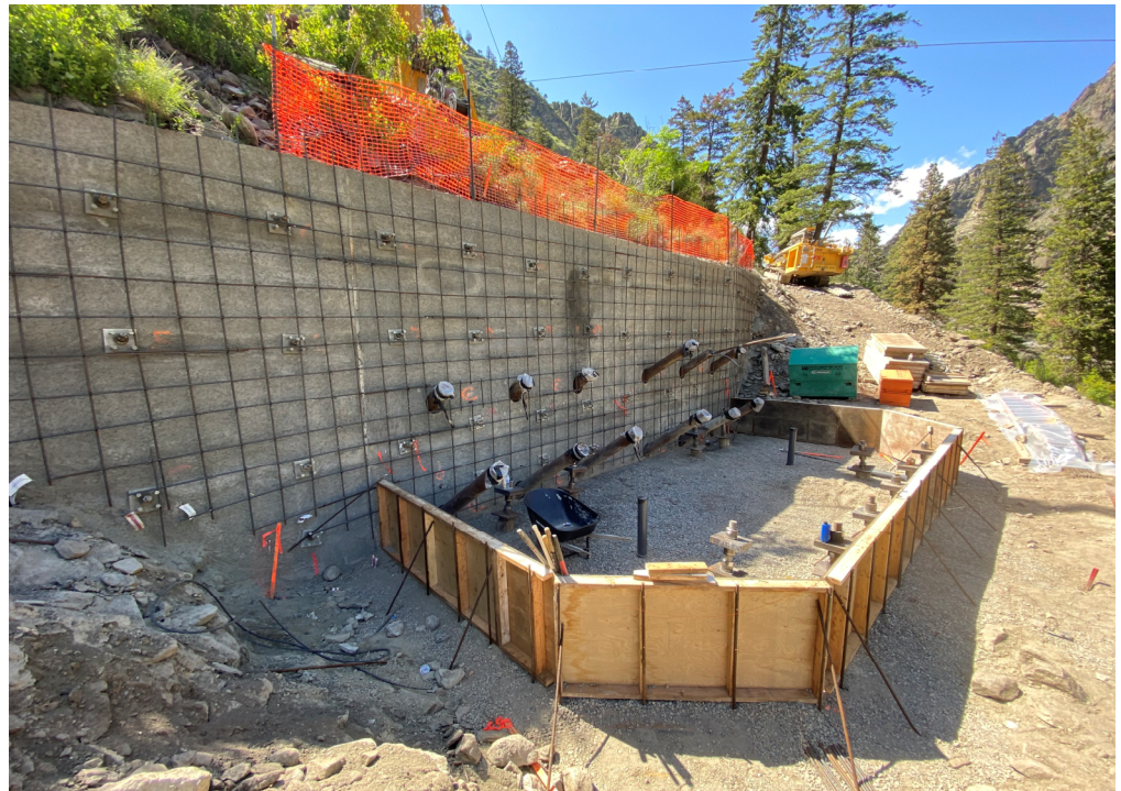
Construction of Abutment 1 facing wall and anchorage
