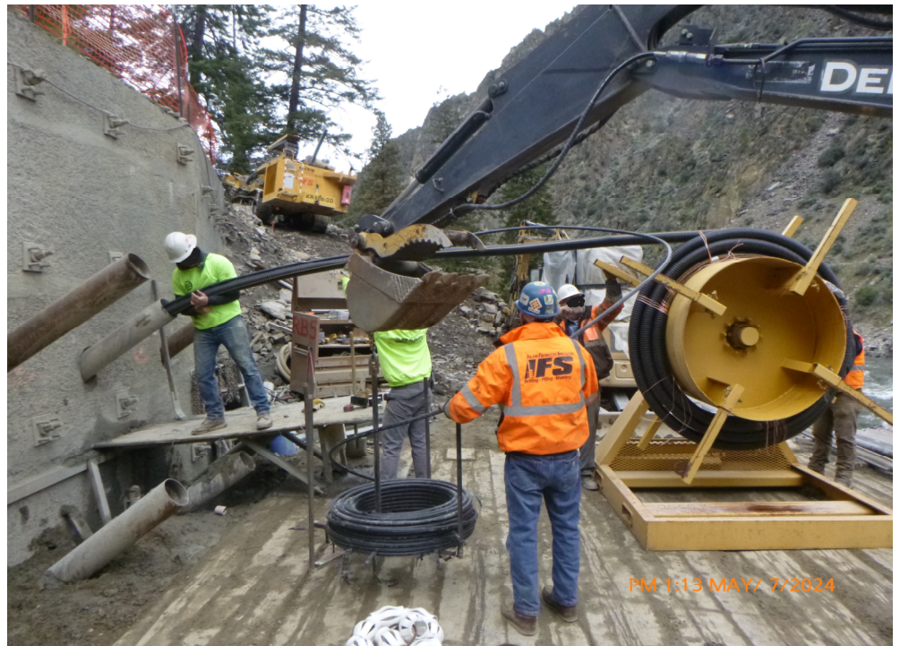
Installing PGA tendon at Abutment 1
