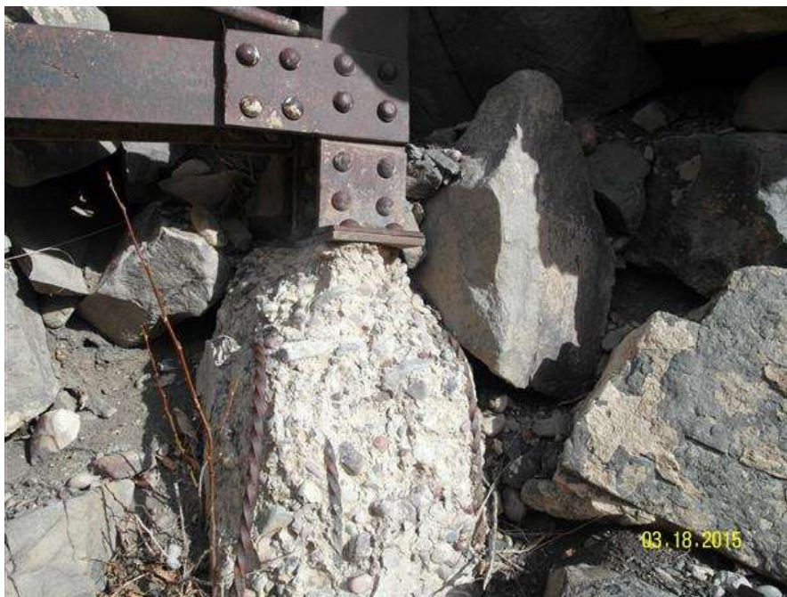
PHOTO #9 MTA-SR-001, SUN RIVER BRIDGE, PHOTO BY GARY GRASSEL. THIS PHOTO IS A CLOSER VIEW OF THE PIER IN PHOTO # 8. (03/18/2015)
