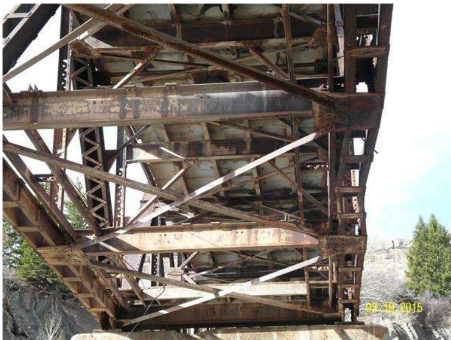
PHOTO #11 MTA-SR-001, SUN RIVER BRIDGE, PHOTO BY GARY GRASSEL. THIS PHOTO SHOWS THE BOTTOM CORD OF THE LEFT UPSTREAM TRUSS. THE BENT LOWER CORD HAS BEEN INSPECTED BY THE RECLAMATION CLIMB TEAM AND NOTHING WAS OBSERVED TO BE IN NEED OF REPAIR. (03/18/2015)
