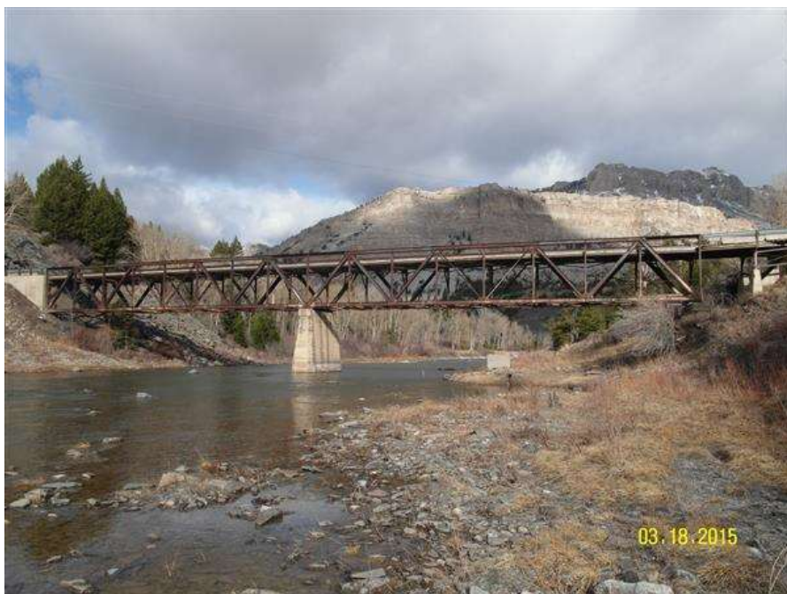
PHOTO #14 MTA-SR-001, SUN RIVER BRIDGE, PHOTO BY GARY GRASSEL. THIS IS A VIEW LOOKING AT THE DOWNSTREAM SIDE OF THE BRIDGE. (03/18/2015)
