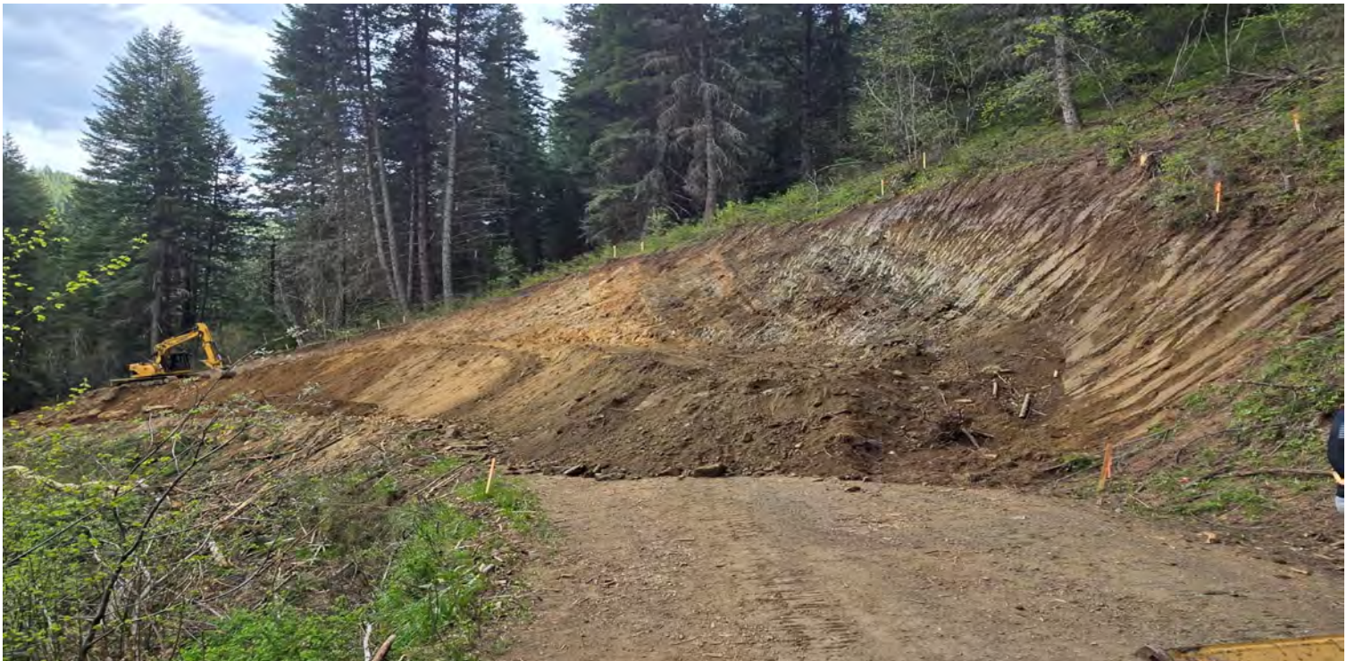
Roadway Excavation at M.P. 13.6
