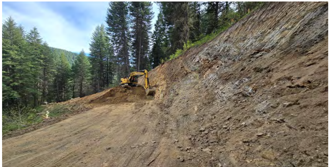
Roadway Excavation M.P. 13.6, FSR354
