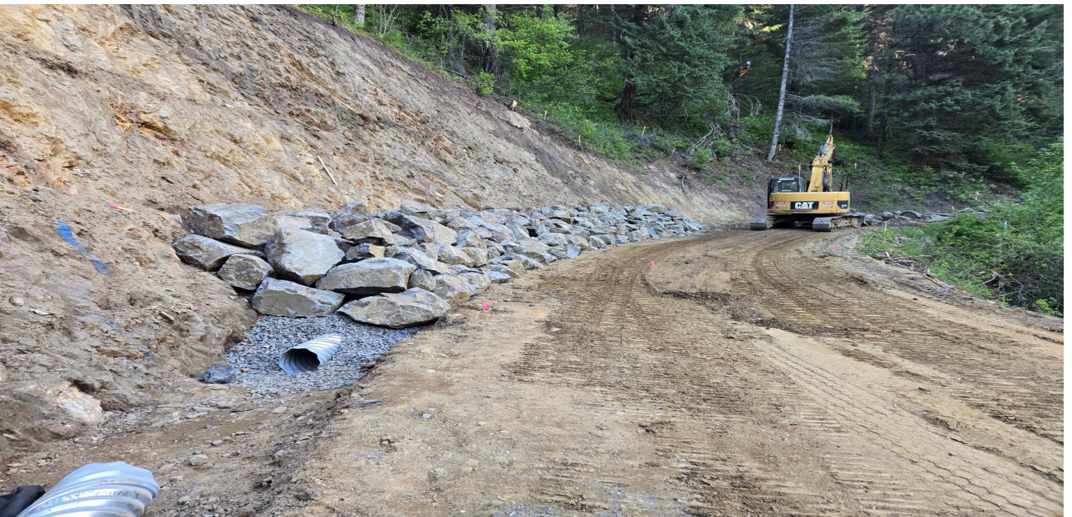
Rock buttress at M.P. 13.6
