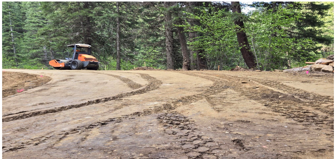
Turnout construction, subgrade prep, M.P. 13.6, FSR354
