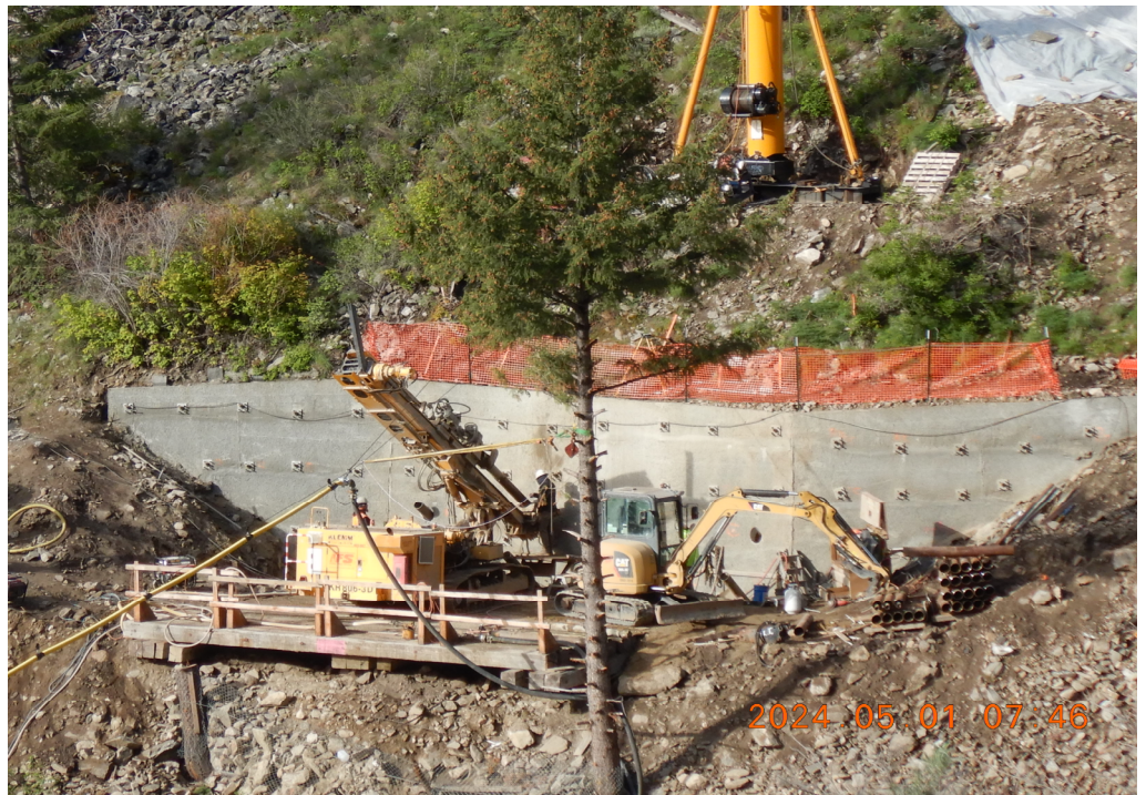
Drilling Permanent Ground Anchor's at Abutment 1
