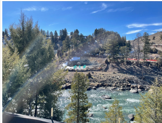
Pier 2 View From Pier 3
