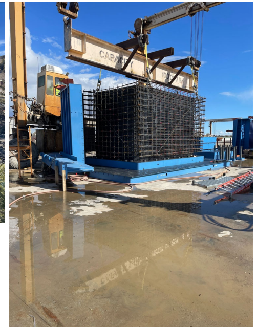
Pier 3 Pre-casting Off-site
