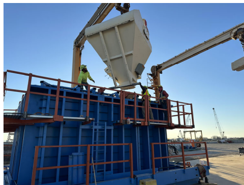
Pier 3 Pre-casting Off-site
