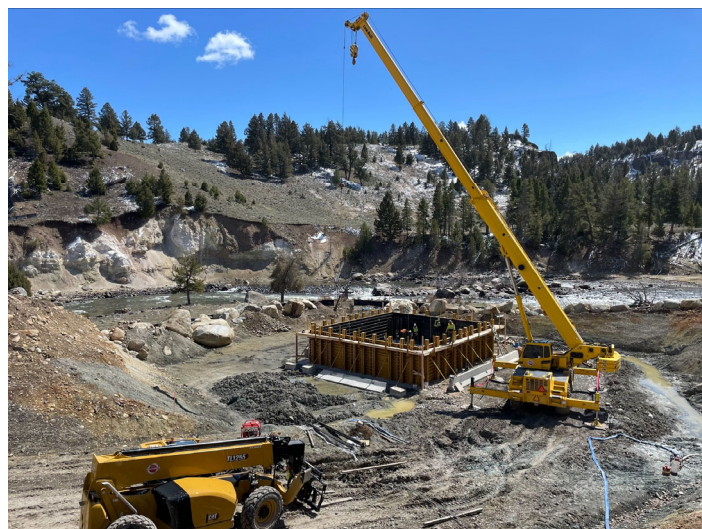
Rebar and Forms at Pier 2
