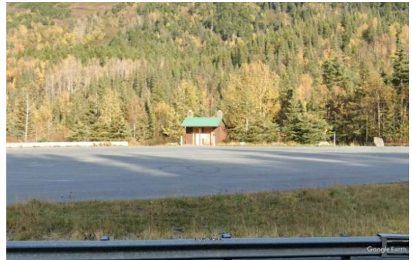
Figure 1-17 Official Rest Area for Turnagain Pass Located at Canyon Creek
