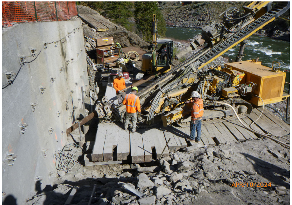
Drilling the ground anchors at abutment 1
