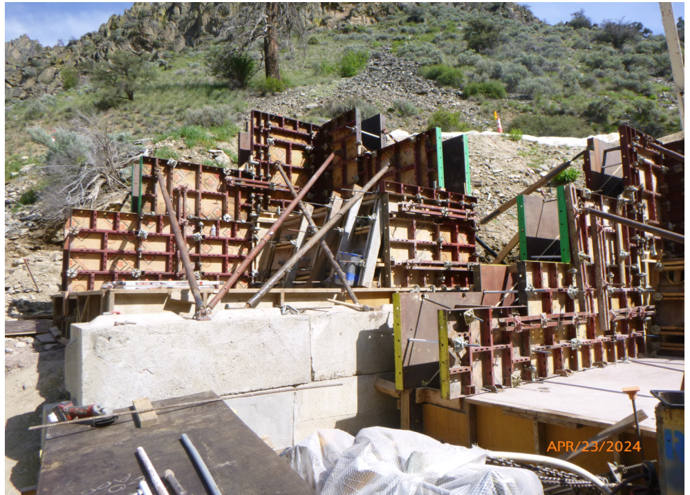
East Anchor Block Formwork
