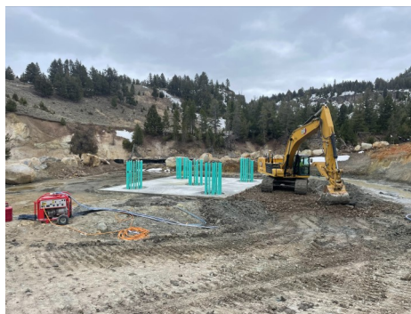
Pier 2 Dewatering and Crane Pad
