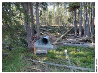
Above: Old Faithful-to-West Thumb culvert installation proceeds in multiple positions along project limits.
