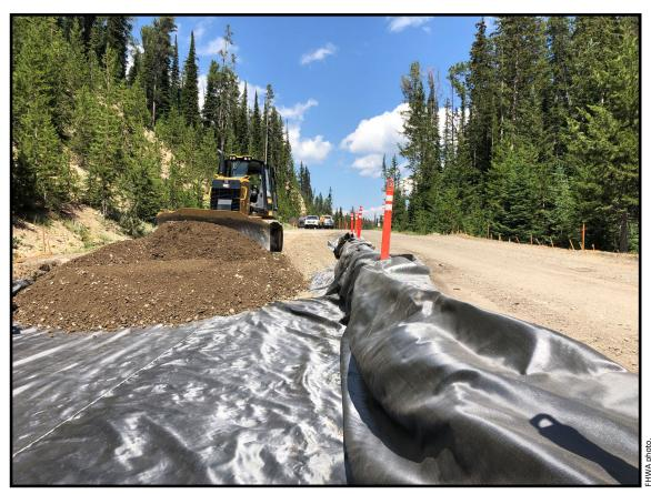
Above: For the Old Faithful-to-West Thumb roadway, geotextile is placed as sub-excavation work proceeds. Continuous one-lane, two-way traffic lanes are maintained daily for tourists, and the park's administrative staff.
