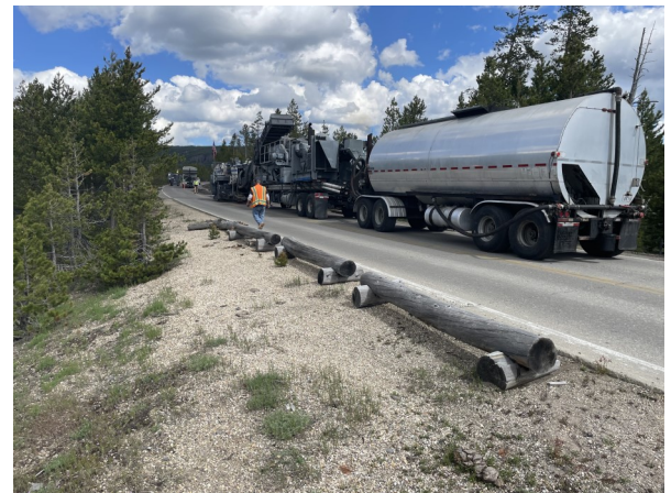
Above: The cold-in place recycle train milling the existing asphalt and creating the new asphalt mix.
