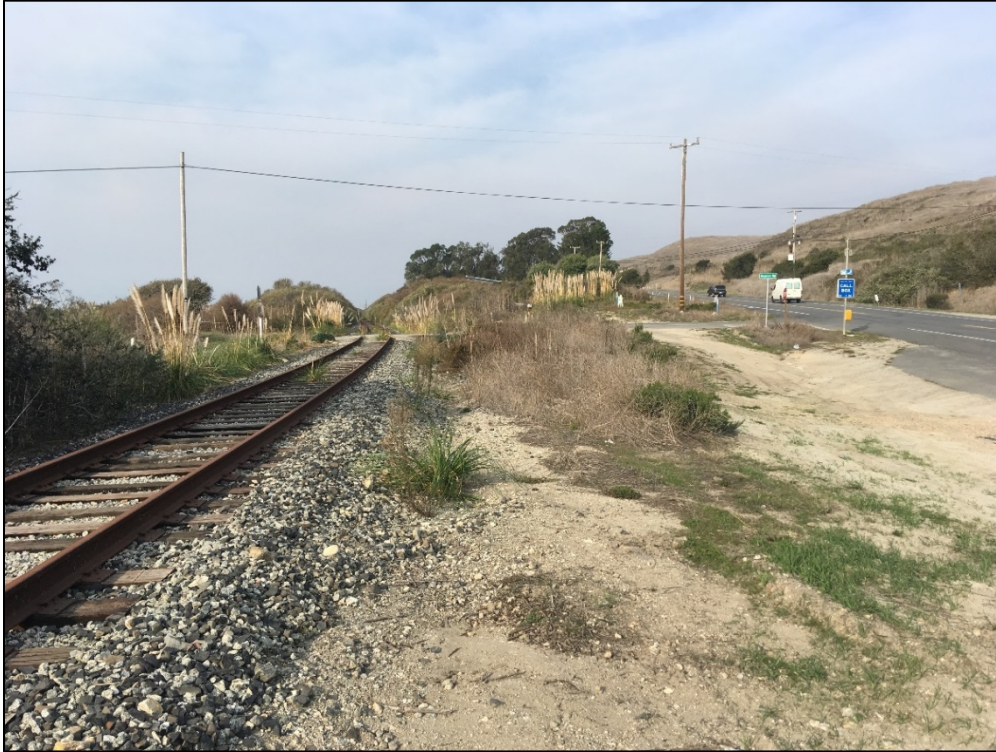
Photograph 5. Rail corridor adjacent to Highway 1 at Scaroni Road crossing, looking northwest
