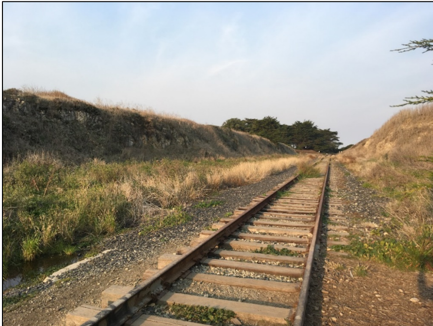
Photograph 2. Northern end of rail corridor below steep embankment, looking northwest
