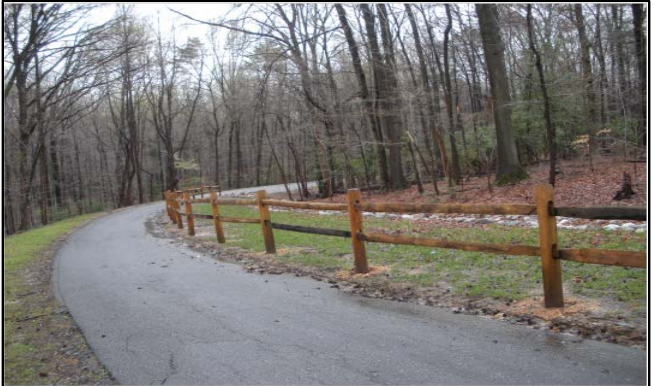
Figure 11. Widen the 250' long section of 9'-7" wide pavement to use as a temporary detour during construction – reset fence at the end of the project & restore to original conditions
