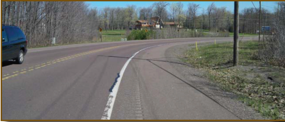
Northbound M-26 (at curve POB)
