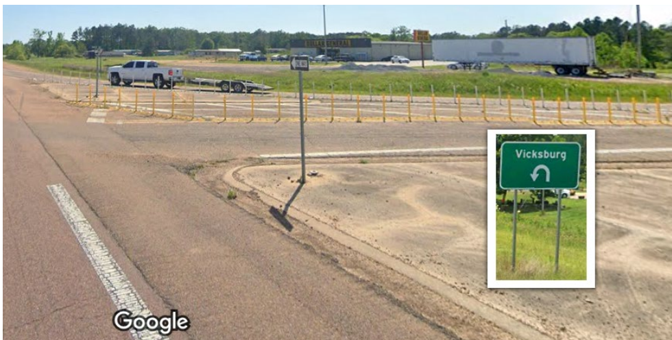
Figure 1. Image. Temporary snap back delineators and supplemental signage were installed on US 533 in Jefferson County, MS to mitigate an urgent intersection crash problem until a permanent RCUT could be installed. Signage was also installed (lower right) to assist drivers in navigating the configuration.
