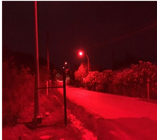
Figure 49. Red LED (610 nm) green turtle-friendly lighting (Image Credit: DMD).
