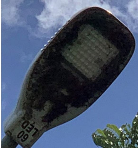
Figure 50. Photo. Rain flies on a luminaire (Image Credit: DMD).
