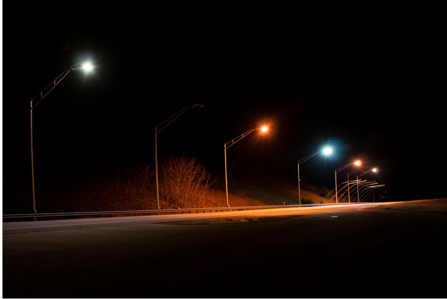
Figure 45. Photo. Photo displaying luminaires of different correlated color temperatures (Image Credit: Rajaram, Bhagavathula, VTTI)
